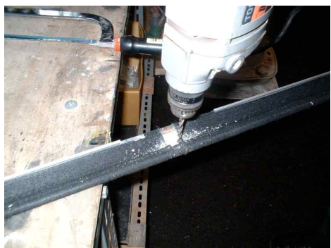
7) After cutting, drill holes.
